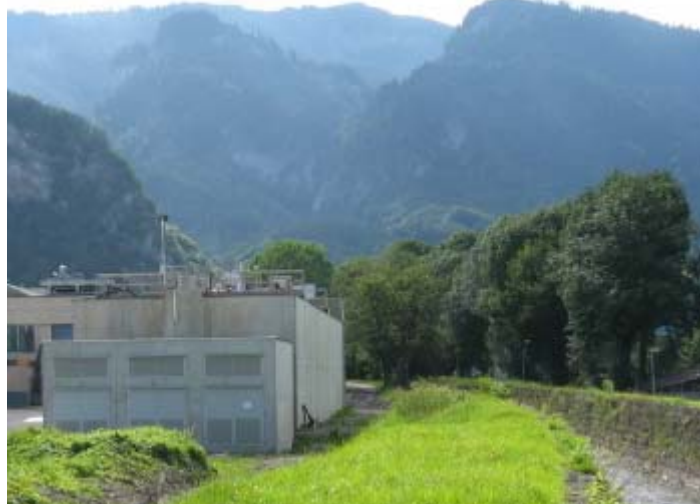
Fig. 1. View of the Collini MBR plant and surroundings.
